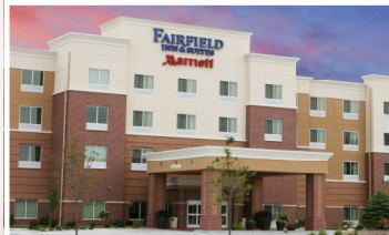
Fairfield Inn & Suites 308-236-4200
